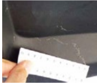
Nail-sensitive scratch or tearing of material. Broken trim or bad repair quality.
